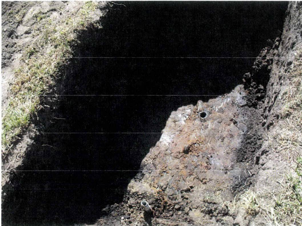
Picture 3: Excavation for UST 768Althea-2.
